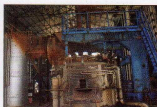
Electric Arc Furnace
